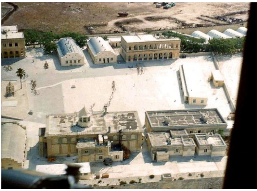
Aerial view of Verdala RN Primary School, Malta around 1960 - playground, classrooms, crocodile of children, palm tree, climbing frame and all!
